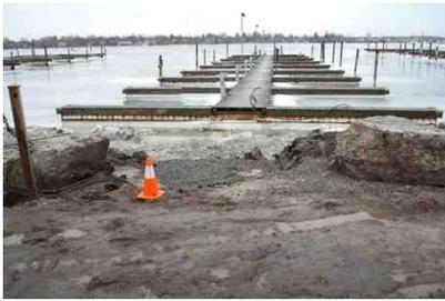
The old concrete base for the ramp to B dock was removed in preparation of an armour stone base. The concrete base had begun to slide into the bay as a result of the old wall failure and last summer's high water.
